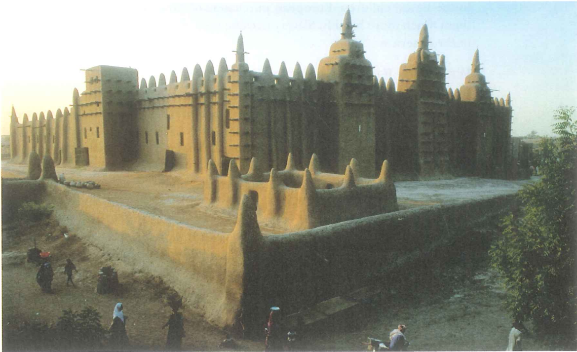
Located in Djenné, Mali, this massive mosque, made of sun-hardened mud, dates from the fourteenth century. At that time, Djenné prospered as a center of trade and Islamic learning.
