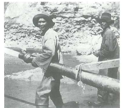
A Chinese mine worker steadies a water cannon in a shallow riverbed in Idaho with a fellow laborer standing nearby.
