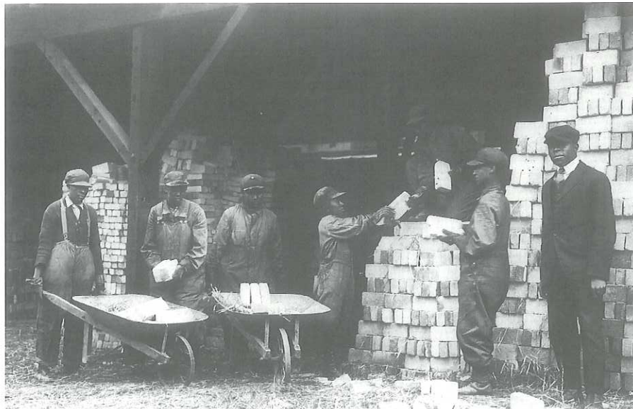
Female workers stack bricks from wheel barrows at a brickyard under the supervision of a man in a suit.
